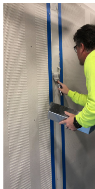
Application of joint compound.
