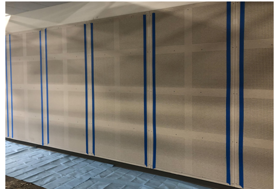
Painters tape applied to perforation field edges.
