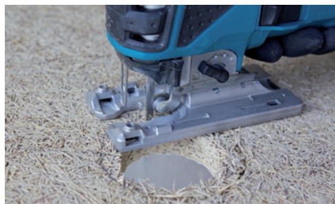
Jigsaw or Hole Saw: Lay the acoustic panel down with the exposed side down. Always make longitudinal cuts with a guide.
