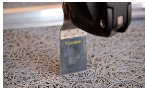
Cutting openings by means of a supercutter Only cut at a right angle to the panel surface.
