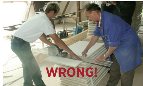
Not this way! Never cut acoustic panels on a stack.
