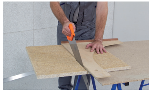
Hand saw: Lay the acoustic panel down with the exposed side up. Always work with a guide. Support the free end of the panel.
