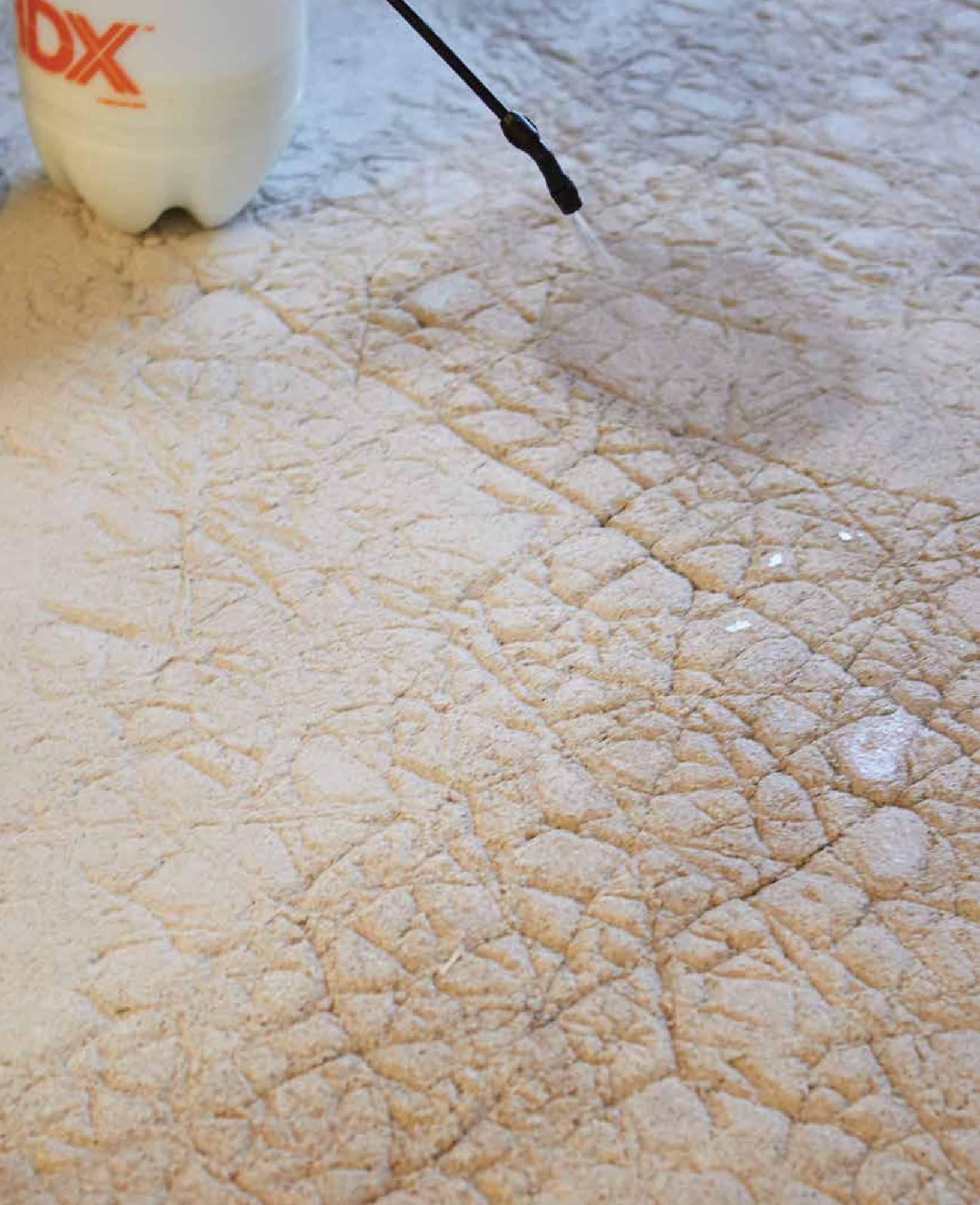
USG Durock™ Fusion™ Primer application over compromised gypsum underlayment.
